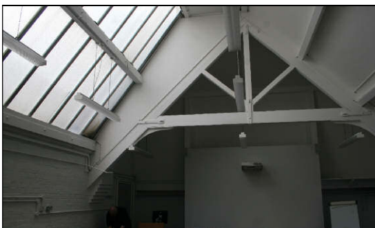
Timber roof trusses in 1883 building
